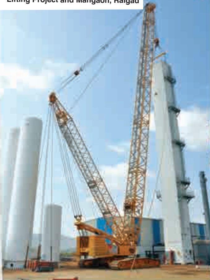
Lifting Project and Mangaon, Raigad
