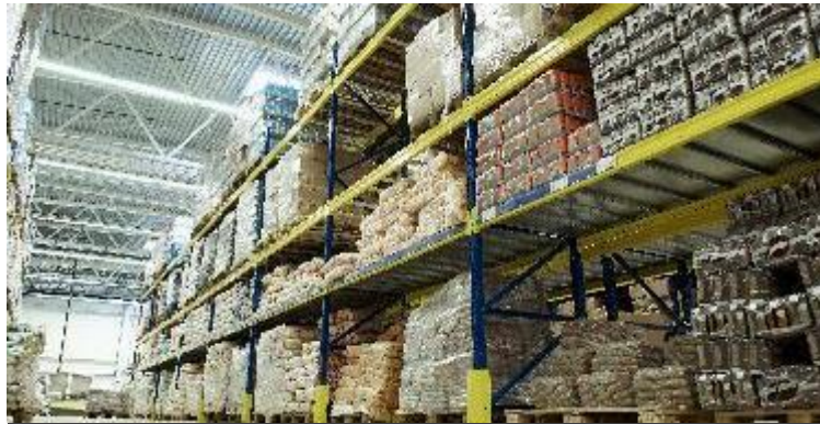
Chemical, Food & Pharma Warehousing
